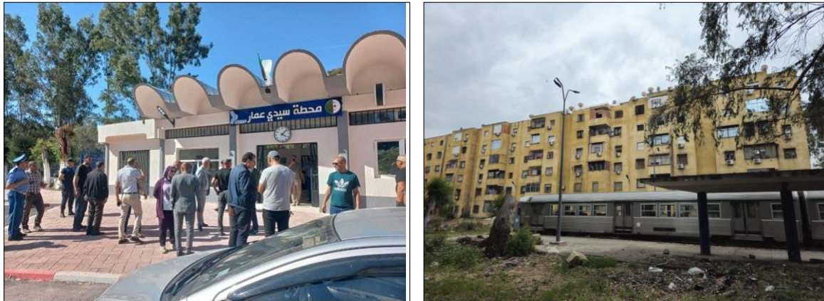
Figure 2. Railway station in the study area.
